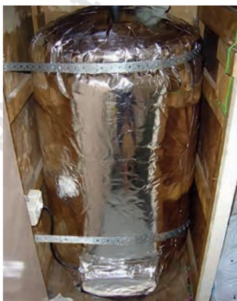
Figure 35 – Insulated hot water cylinder
