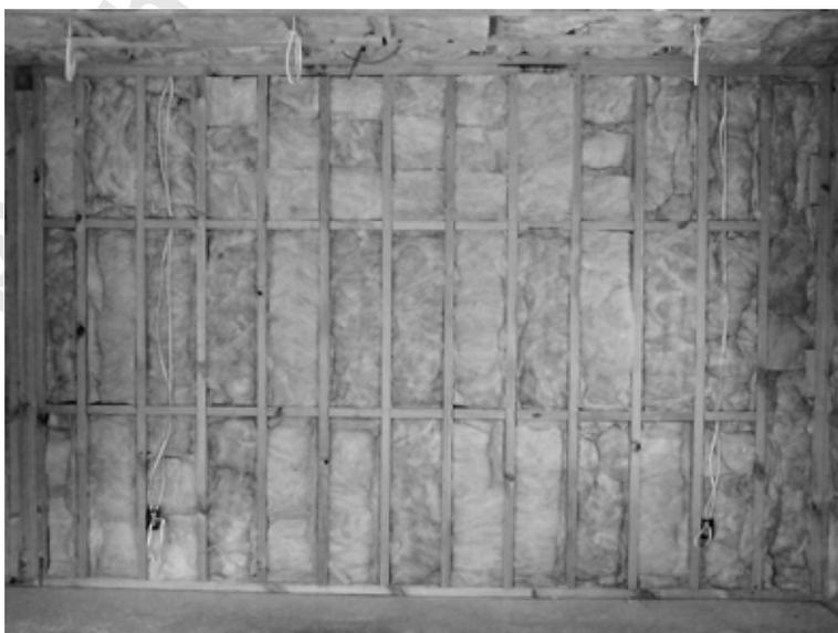
Figure 1 – Insulation installed with gaps, tucks and folds
