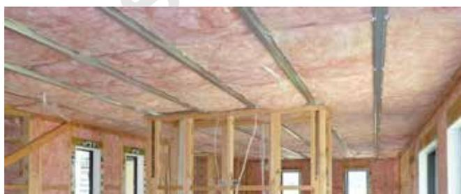
Figure 27 – Segments installed in a ceiling
