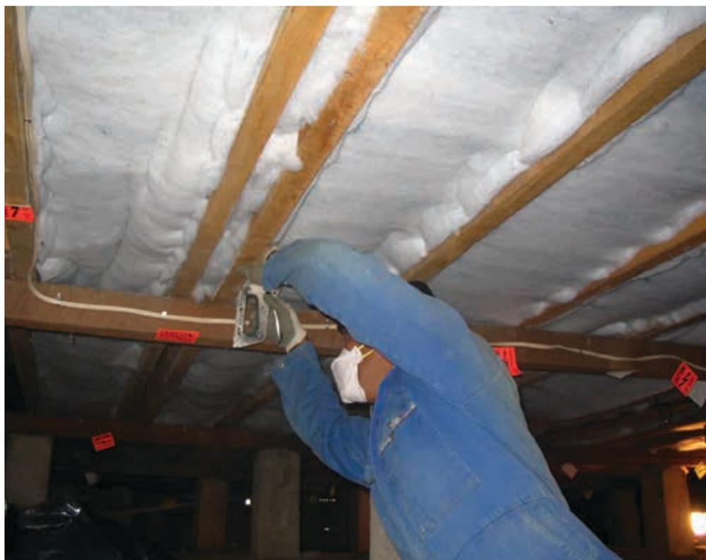
Figure 30 – Installed underfloor blanket
