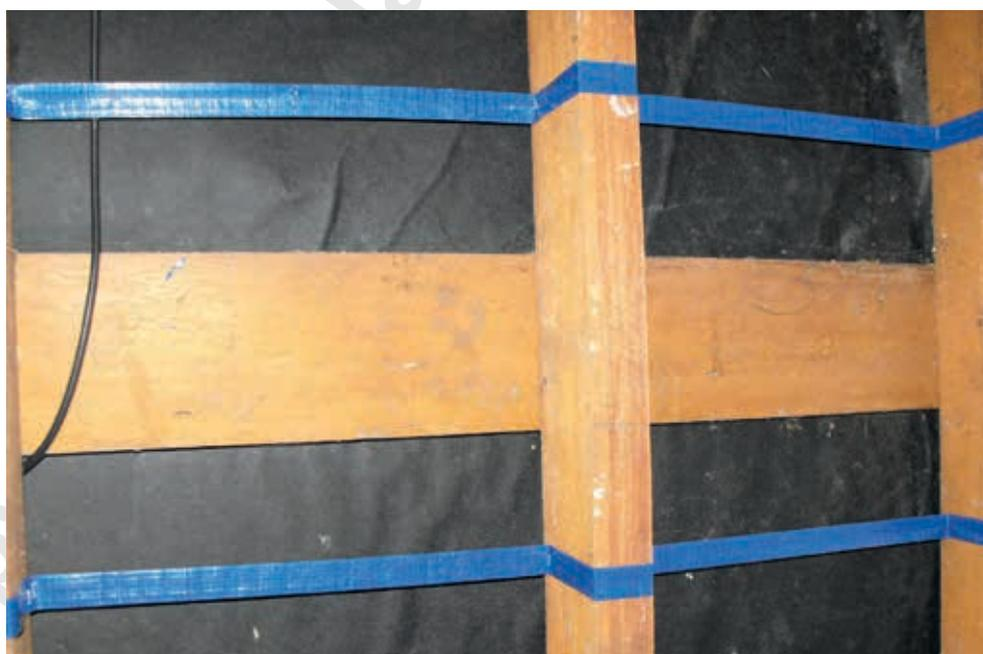
NOTE – The figure illustrates the way of strapping the wall before insulation is retrofitted in walls without wall underlay (Method 1). Ignore the wall underlay shown in the photo.
