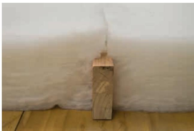
Figure 29 – Friction-fitting insulation over joists
