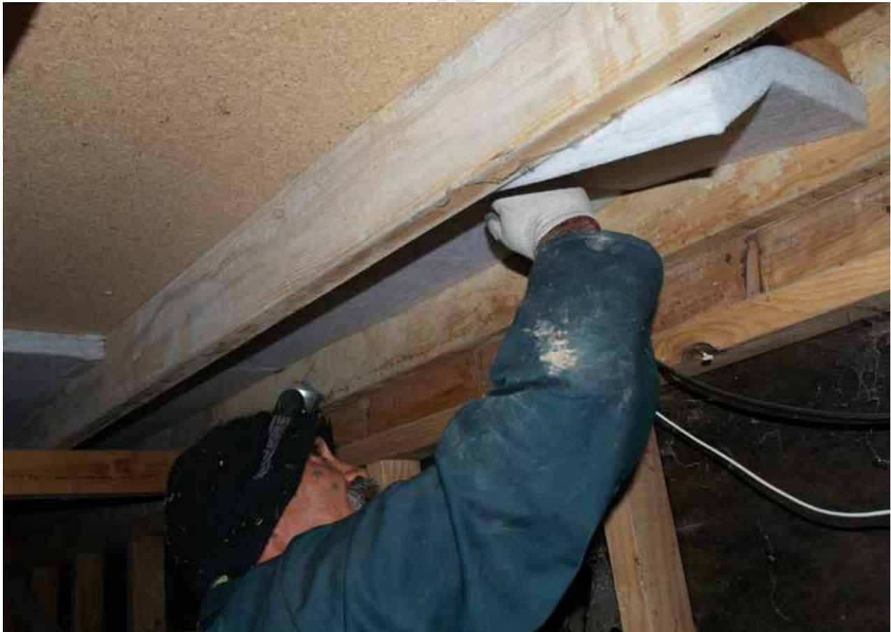
Figure 32 – Fitting semi-rigid sheets
