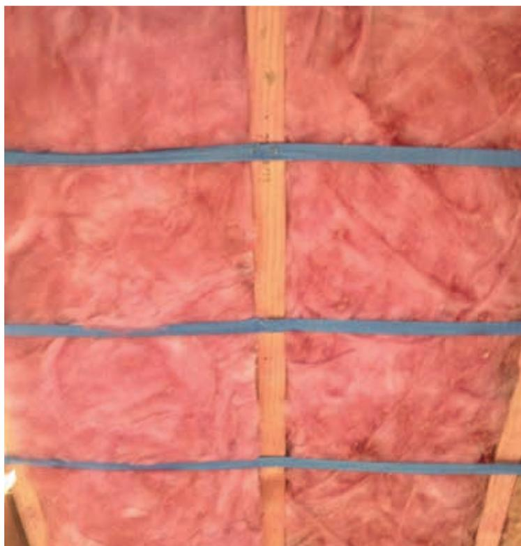
Figure 28 – Blanket in a ceiling secured with strapping
