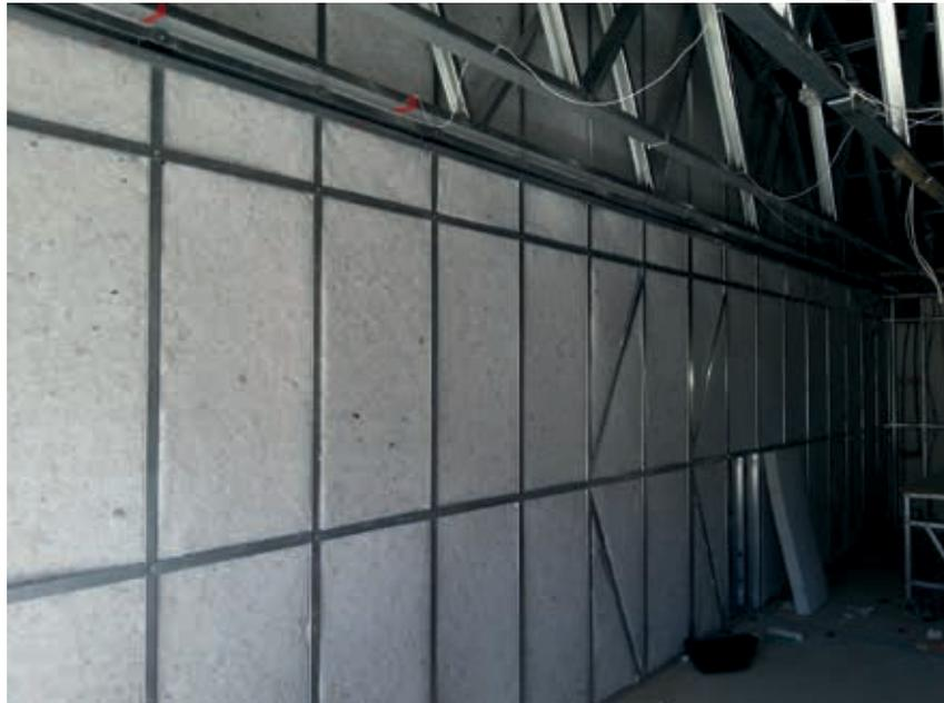
Figure 16 – Insulation fitted into a steel-framed wall
